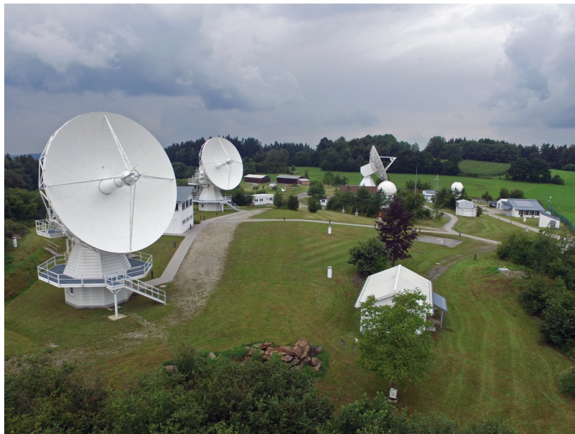
Figure 30: The Geodetic Observatory Wettzell with the two 13.2 m TWIN radio telescope antennas in the foreground on the left and the 20 m Radio Telescope Wettzell in the background on the right.
