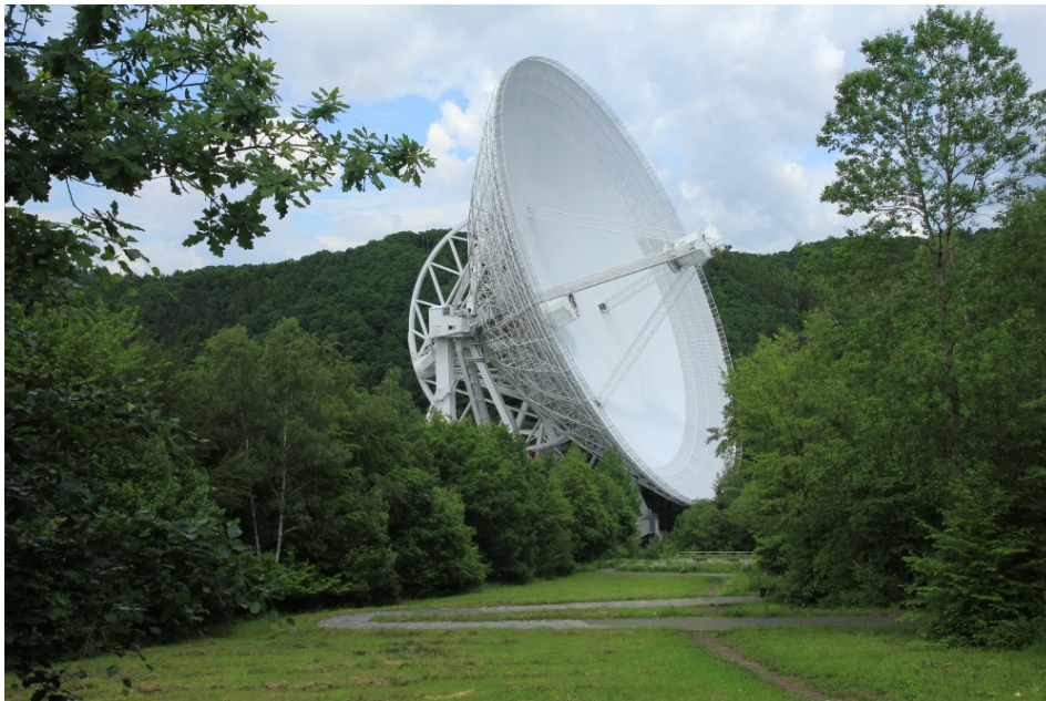
Figure 16: The Effelsberg 100m radio telescope as seen from the public visitors pavilion in Autumn 2016. The main dish panels were freshly painted during the maintenance periods in summer 2015 and 2016. (photo N. Junkes, MPIfR)
